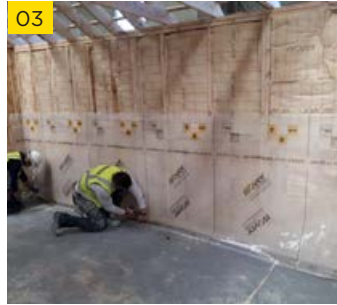
03 Apply Vario KM Duplex or Vario Xtra across/along the studs using a staple to secure the membrane in place.
