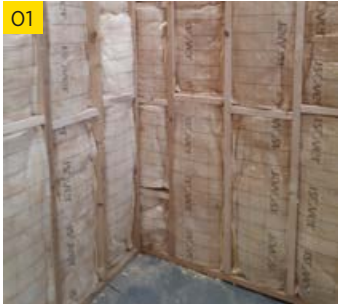
01 Cut & friction fit ISOVER Metac O31/O34 Insulation between studs/rafters.
