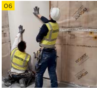
06 Install the first board at the corner of the knee wall, ensuring a snug fit. Ensure the edge of the board has adequate support from the vertical framing timbers, splitting each joint stud between the respective InLiner Boards.
