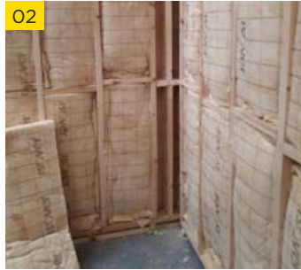
02 Ensure that suitable timber grounds are located to support InLiner boarding perimeters.
